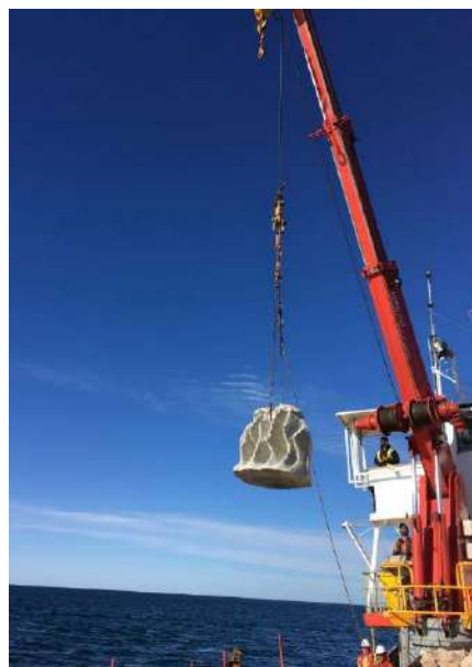
One of the custom made concrete structures for oyster reef reconstruction being lowered into place on the new reef (PIRSA)
